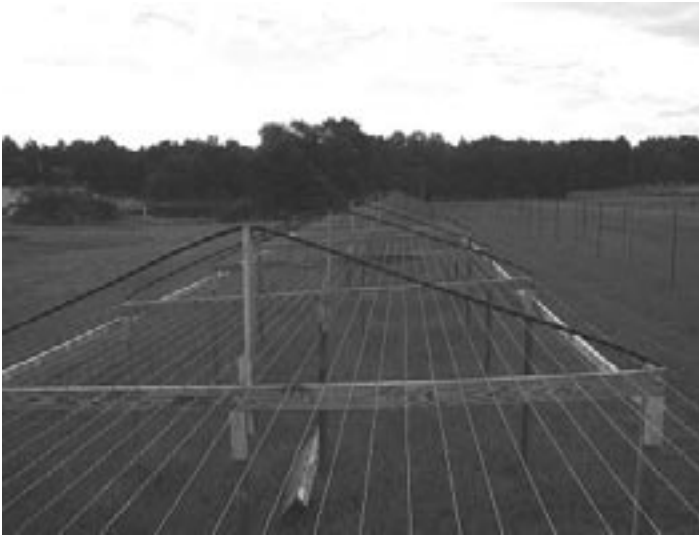
Figure 15-5. High-tensile-wire curing structure
